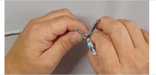
Roll back the braid or drain wire onto cable so it is out of the Separate the four pairs and remove the foil wrap from around each pair.
