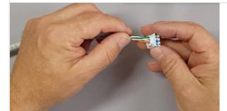
Insert the wires through the back of the wire forming cap
