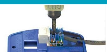
With twists right up to the IDC terminals, use 110 Tool to terminate
