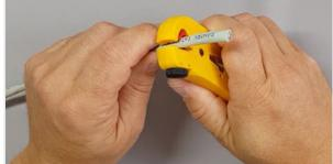
Strip 40mm of sheath from cable using stripper
