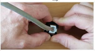
Continue to press down on outer clamps until they are fully closed. This will ensure the terminations are complete.
