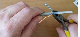
Remove the inner divider and stripping braid
