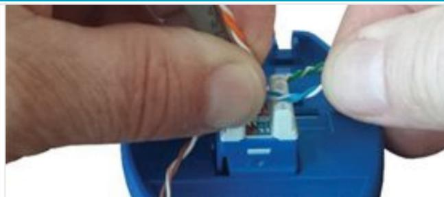
Using working base, place wires as per color spec
